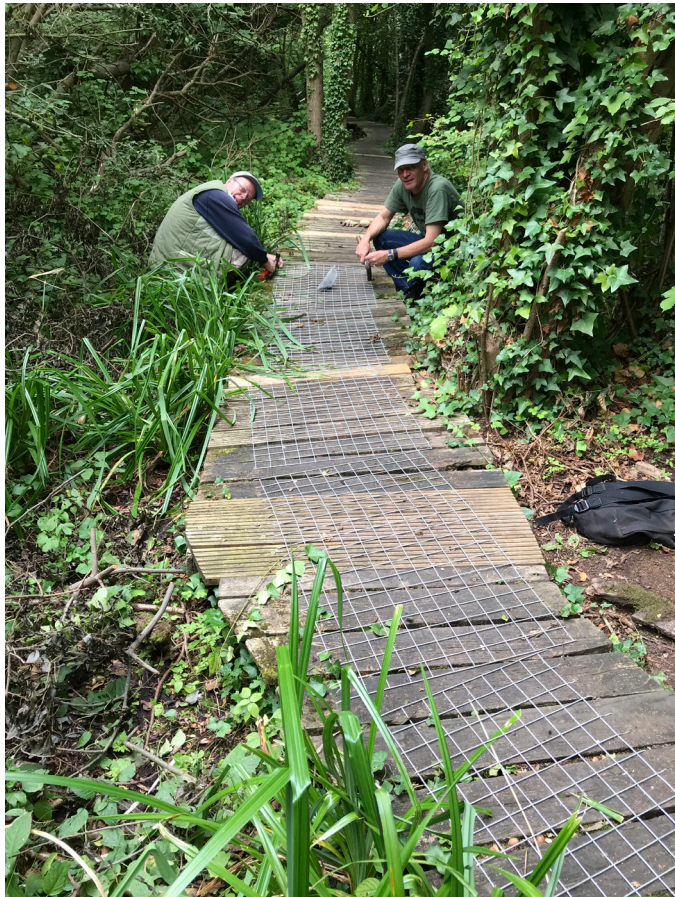
Repairing boardwalks and bridges
